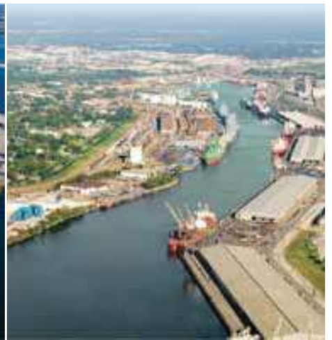
Port of Houston Authority Project 11 Ship Channel Expansion.
